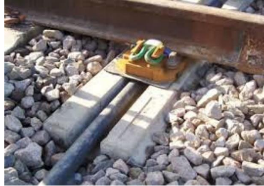
Plate 1. Concrete hollow sleepers
